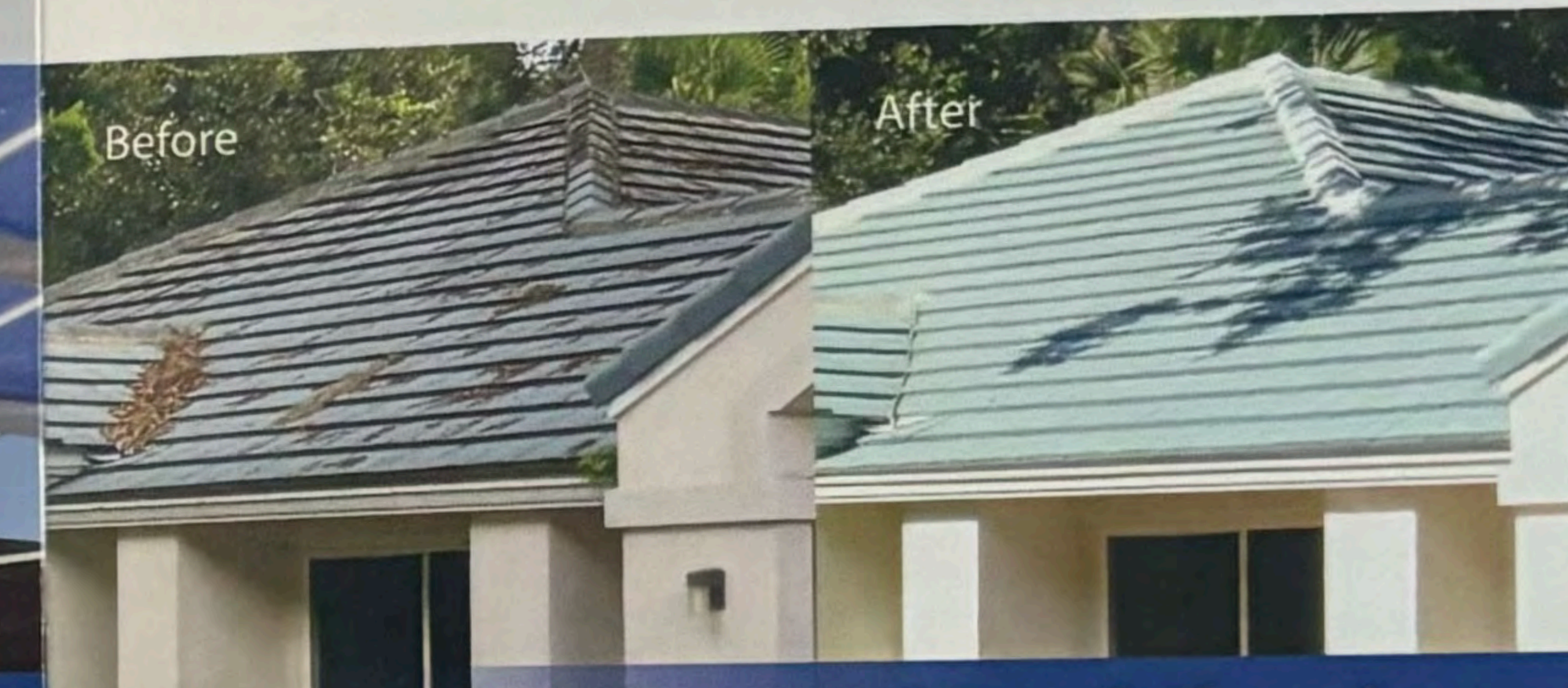
Commercial Roof Cleaning
