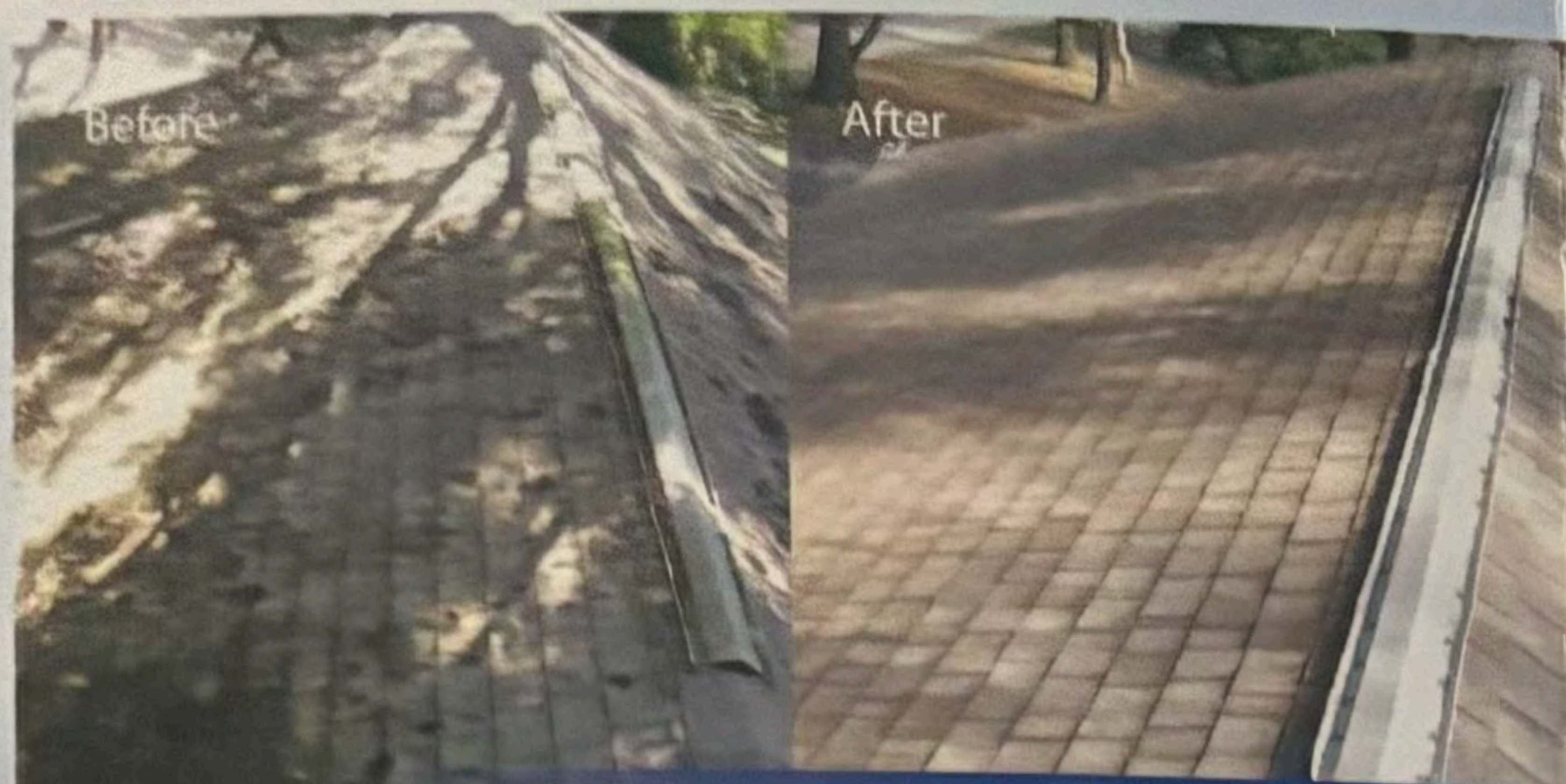
Low Pressure Roof Cleaning
