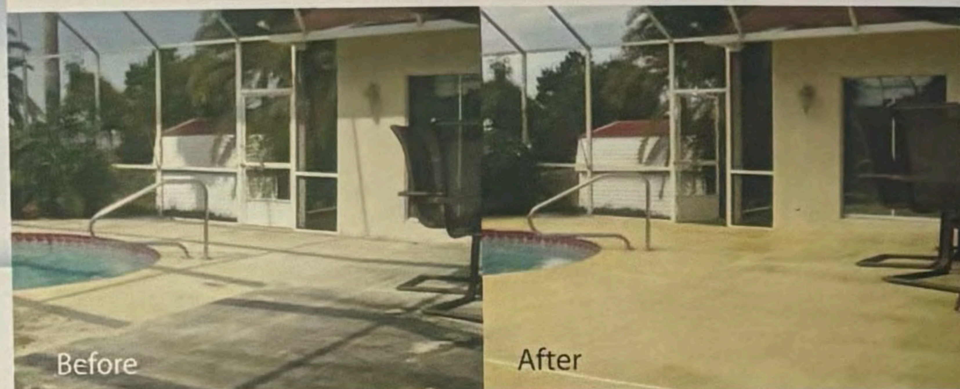
Concrete & Brick Cleaning
